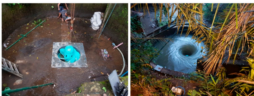
Figure 58. Installation with winch (left) and manual lifting (right) first test run.
