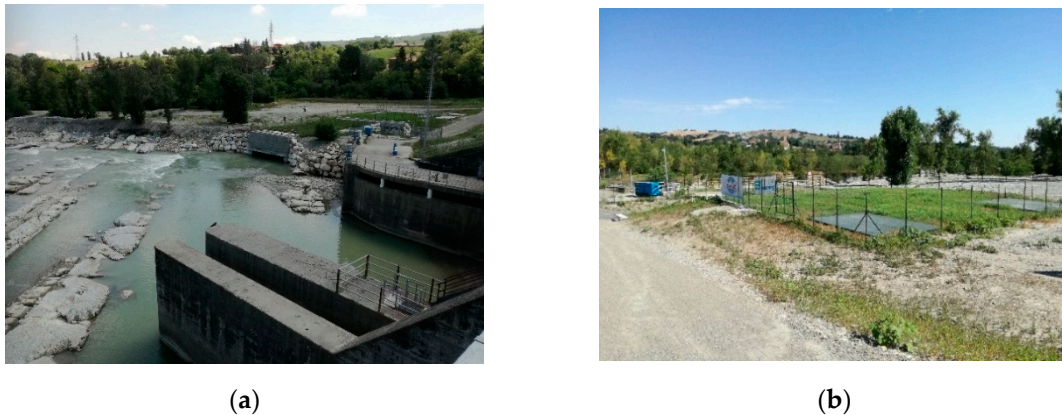
Figure 32. (a) photo from the upper side of the weir; (b) photographic shooting of the access to the building.
