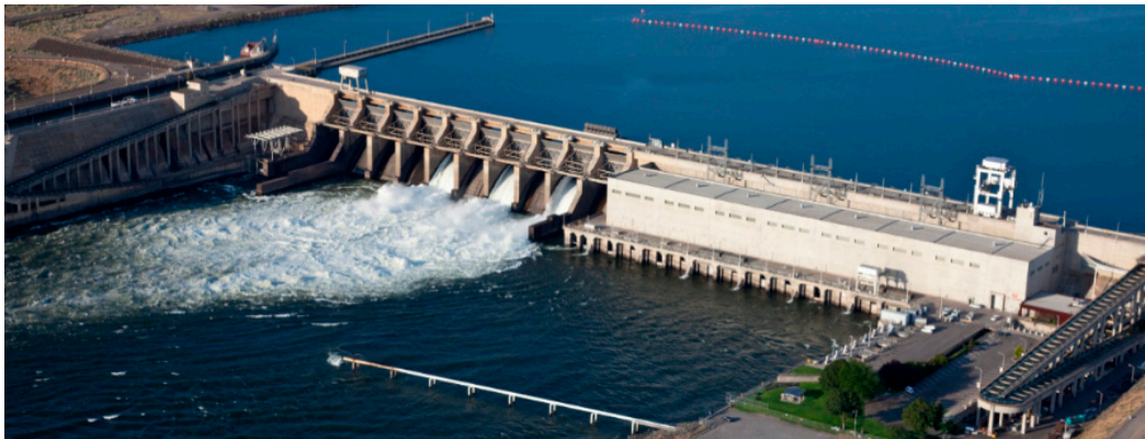
Figure 22. Ice Harbor Lock and Dam, located on the Snake River in southeast Washington State, U.S.
