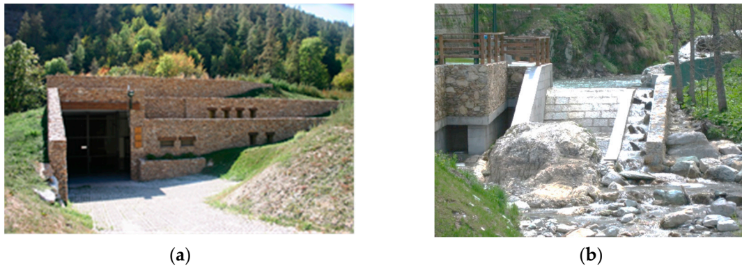
Figure 24. HPP “Frere 2”—Powerhouse (a) and intake works with the fish ladder (b).
