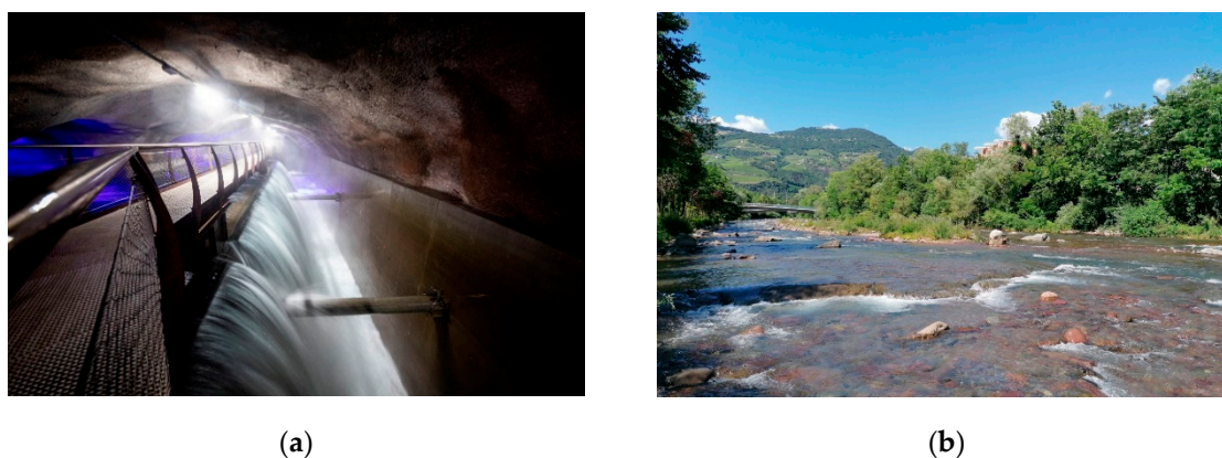
Figure 18. (a) The underground demodulation reservoir built at the S. Antonio plant in Bolzano, Italy. It was built between 2016–2018 and has a maximum capacity of approximately 95,000 m 3 . (b) View of the Talvera river downstream of the power plant.
