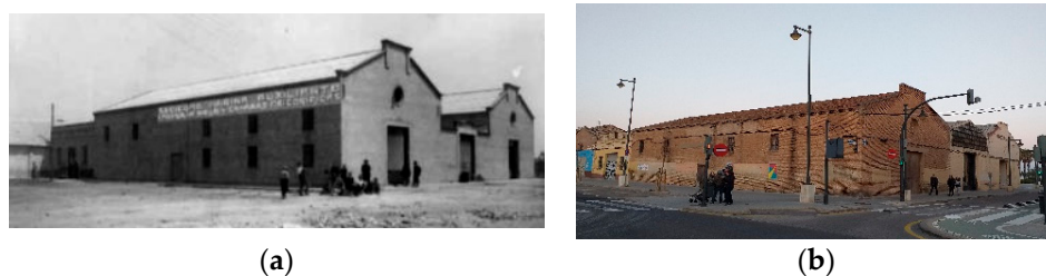
Figure 8. Photo of the Fábrica de Hielo: (a) Historical photo taken between 1931 and 1950 [27,28]; (b) current photo 2019.
