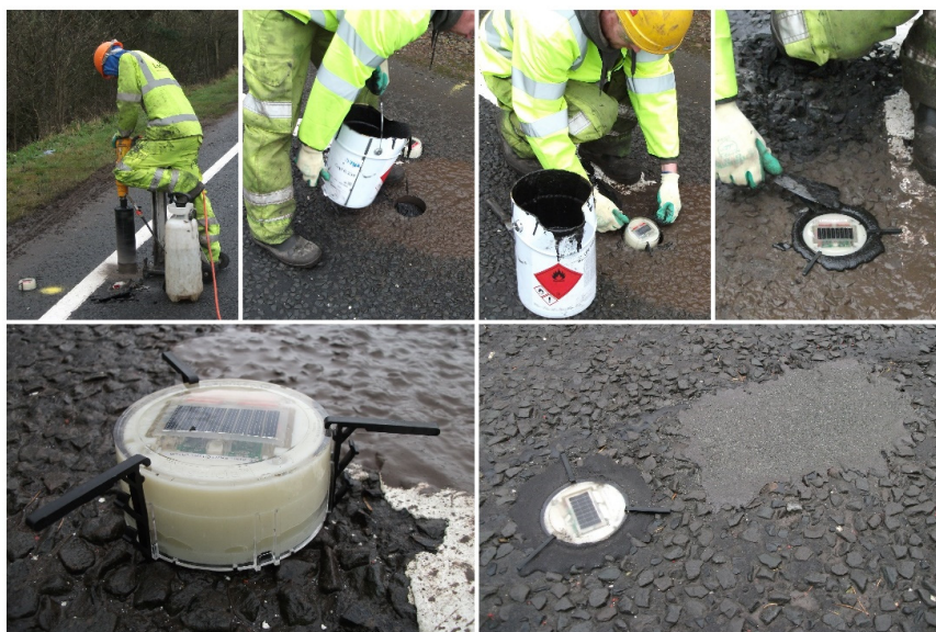
Figure 1. Installation process for the active road stud.
