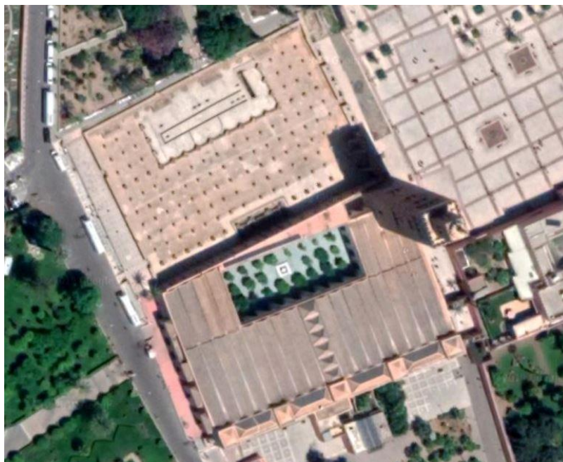
Figure 1. Koutoubia mosque architecture. Source: Google Maps.
