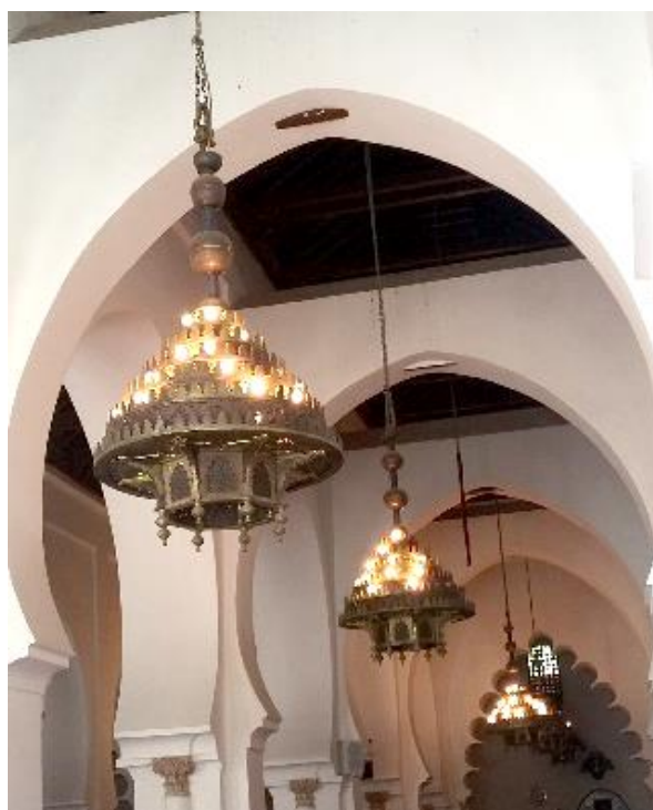
Figure 8. Photo of the chandeliers containing incandescent lamps before revamping with LED lamps.
