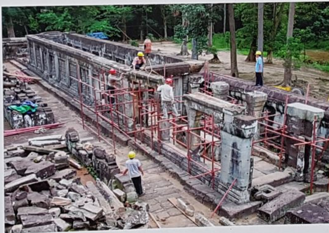
修复中 During Restoration
