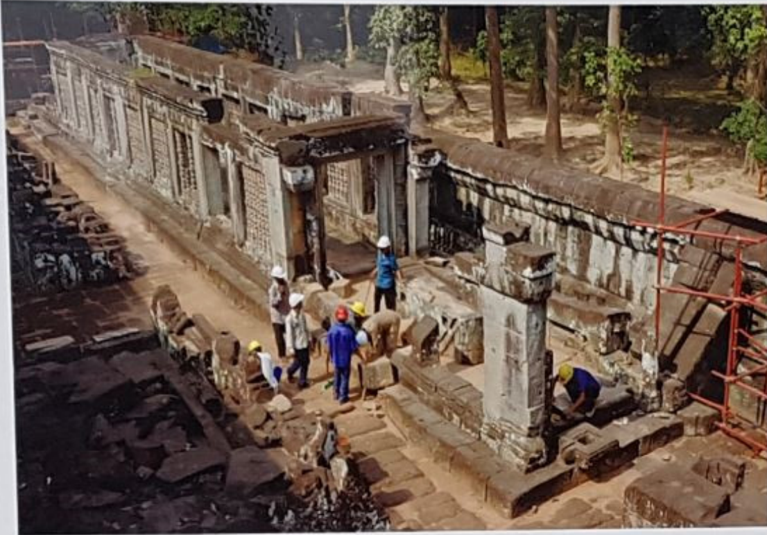
修复中 During Restoration
