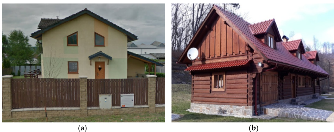
Figure 1. Views of the assessed wooden family houses: (a) wooden frame house; (b) log house.
