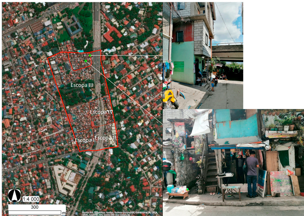
Figure 4. Site Impression of Barangay Escopa in Quezon City. (Above right) ISFs in the Oval Area of Escopa III next to Katipunan Avenue very prone to landslide. (Below right) haphazard housing conditions in Oval Area. Source: own illustration based on GIS base map 2020 and authors' field visit photos in February 2020.
