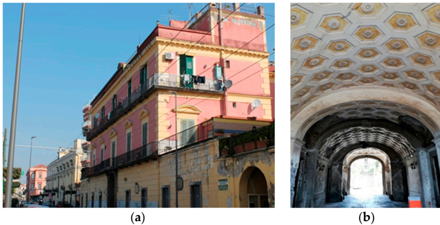
Figure 4. Villa Arena: main facade (a) and entrance hall (b).
