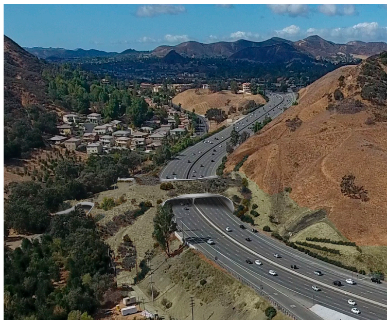
Figure 1. Rendering of a proposed Liberty Canyon wildlife crossing structure over Interstate 101, Los Angeles County, California. The proposed crossing will span 10 lanes of traffic. Photo credit: Resource Conservation District, Santa Monica Mountains, Clark Stevens Architect, Raymond Garcia Illustrator.
