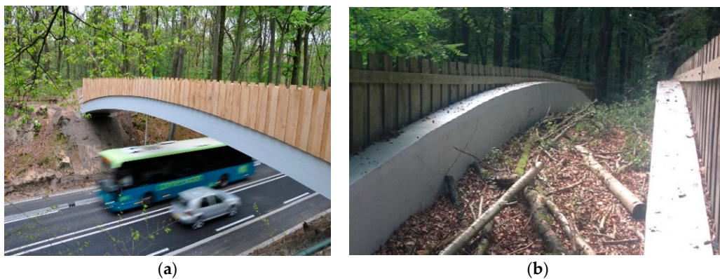
Figure 6. Example of vacuum assisted resin transfer FRP bridge in Rhenen, The Netherlands. This overpass on the N-225 highway is the first FRP structure designed for wildlife use. (a) The bridge dimensions are 24 m × 2 m. Photo credit: FiberCore Europe. (b) The top of the structure provides a wildlife-friendly surface. It is covered with topsoil and biomass, including plant material used from the surrounding area. Photo credit: Matthew Bell.
