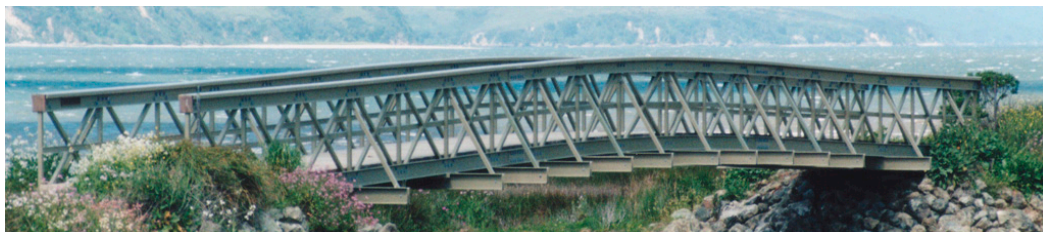
Figure 4. Example of pultrusion-style pedestrian bridge in Marshall, CA. The bridge spans 29 m and is 1.8 m in width. With a live-load design of 2.83 kilopascals (kPa), or 60 pounds per square-foot (psf), the FRP members are connected with galvanized steel bolts. Photo credit: Creative Pultrusions, Inc.
