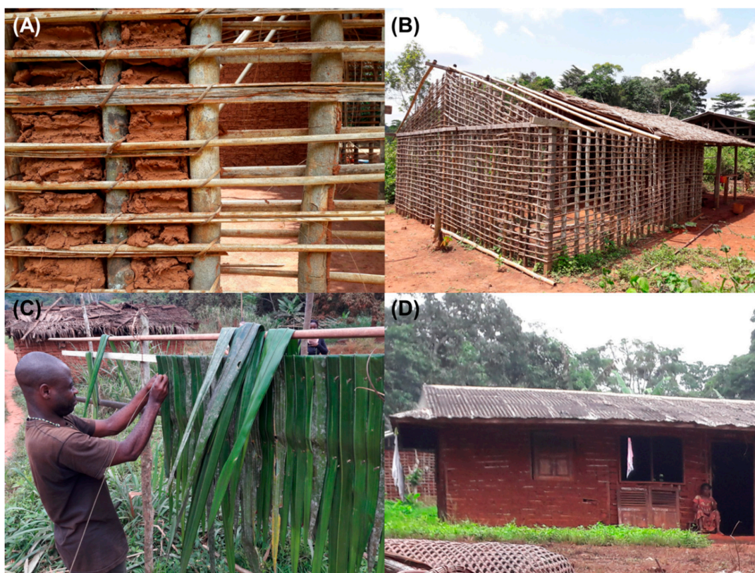
Figure 3. Traditional house type considered for the estimation of timber use in the integrated assessment of ecosystem services use in three villages (Dja area, southeastern Cameroon). (A,B) Traditional house structure. (C) Making of straw roof. (D) Roof plate.
