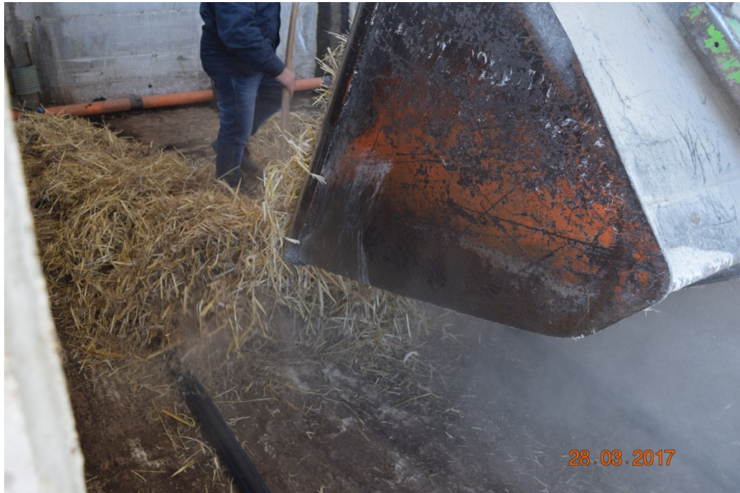
Figure 4. The composting mixture placing on the ventilation pipes.
