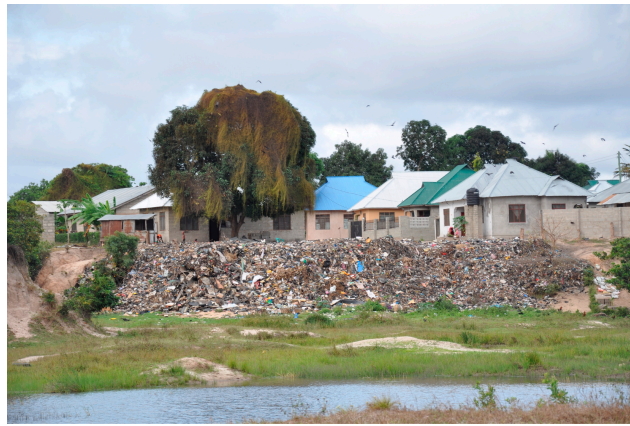
Figure 15. A flood embankment constructed using living garbage, Chamazi.
