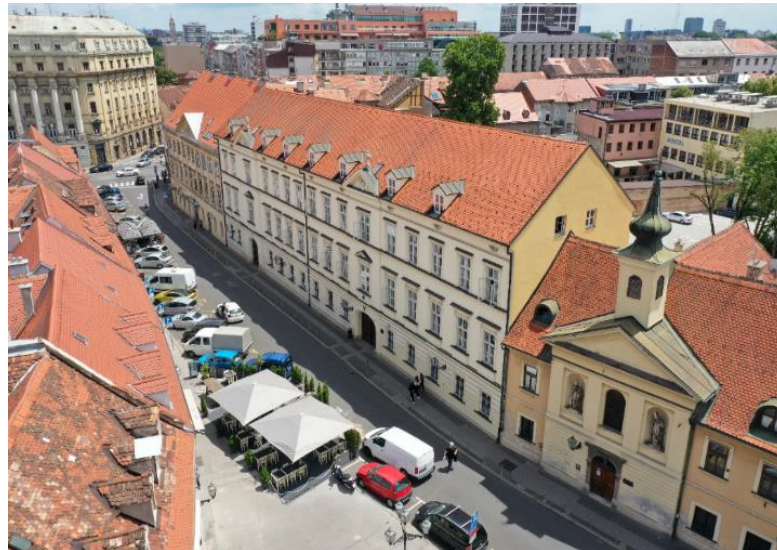
Figure 4. Aerial view of the building—north façade (photo credit: M. Stepinac).
