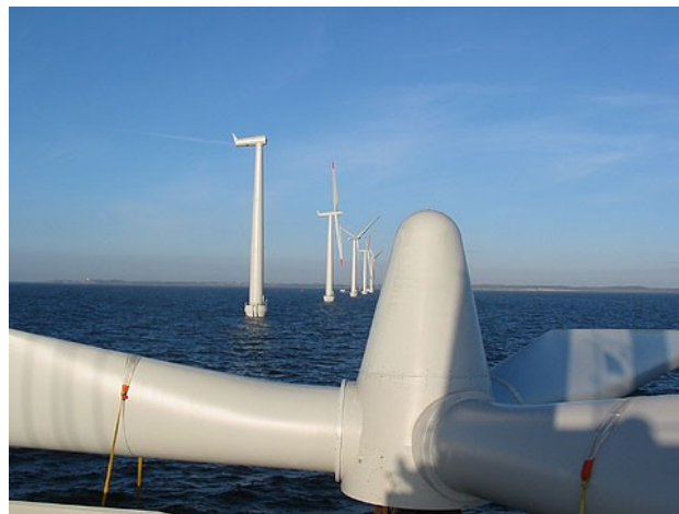
Figure 8. Samsø Renewable Island, Denmark. Source: Soren Hermansen.
