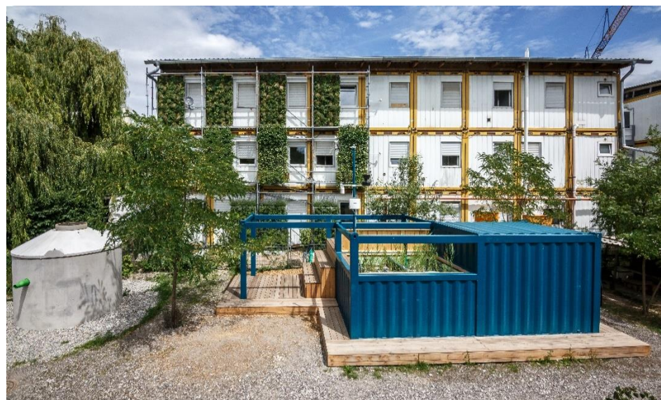
Figure 10. The Impulse Project in built state. On the left: retention cistern made of reinforced concrete with throttled emergency overflow. On the right: two container frames with integrated constructed wetland. In the background: façade greening on residential containers. Rainwater is directed from the roof into the cistern. Grey water is available from the sanitary containers (far right in the picture). Photo: Julian Rettig.
