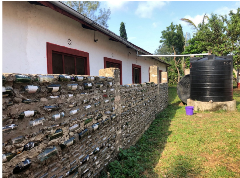
Figure 3. Maendeleo Academies: Rainwater catchment tank and wall built with recycled glass bottles.
