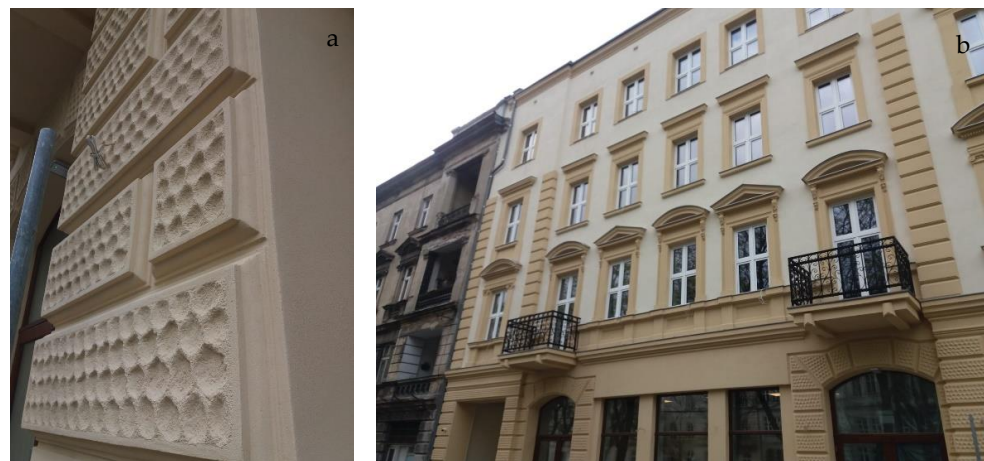
Figure 5. (a) Fragment of reconstructed rustication on the facade 29 April 2021; (b) tenement house after refurbishment 29 April 2021, authors' archive.
