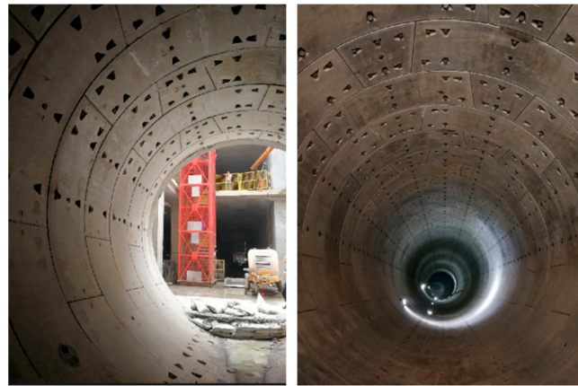
Figure 9. Site photographs of rail transit tunnel Line 3 in Jinan.
