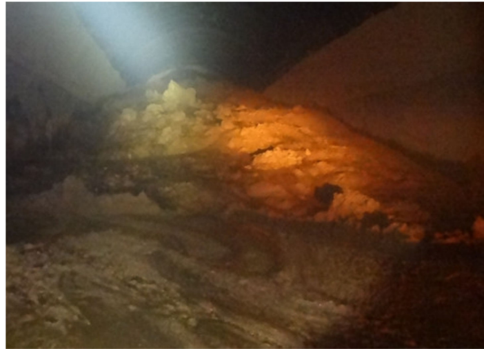
Figure 6. Inrush in right tunnel for the third time.
