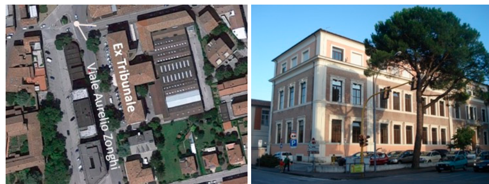
Figure 1. View of the case study building.
