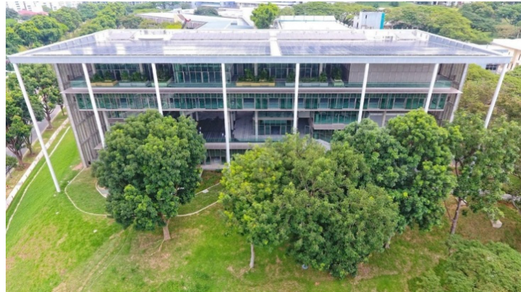
Figure 5. Singapore's first 5G-enabled NZE building in NUS.
