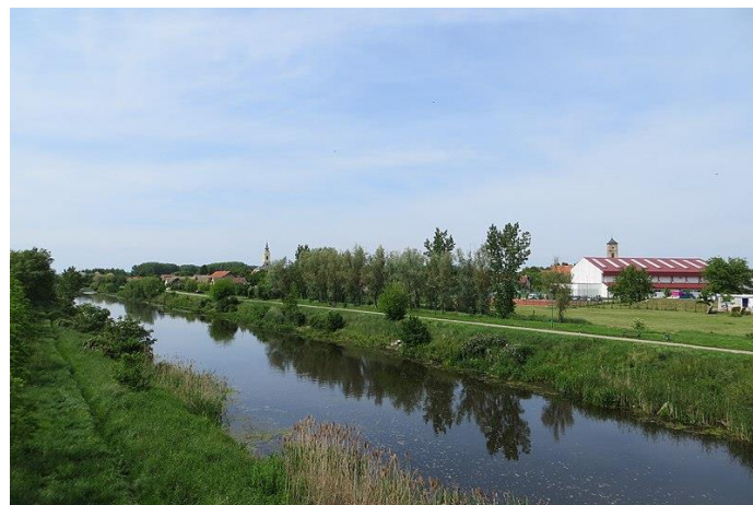
Figure 3. Canal Karavukovo Backi Petrovac. (source https://commons.wikimedia.org/wiki/File:Kanal_Karavukovo-Ba%C4%8Dki_Petrovac_-_panoramio.jpg (accessed on 13 June 2021)).
