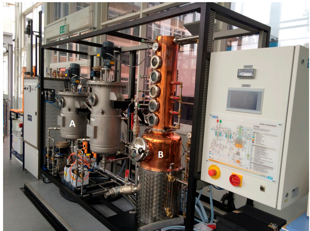
Figure 1. Extraction facility—(A) Extraction tank and (B) Distillation column.
