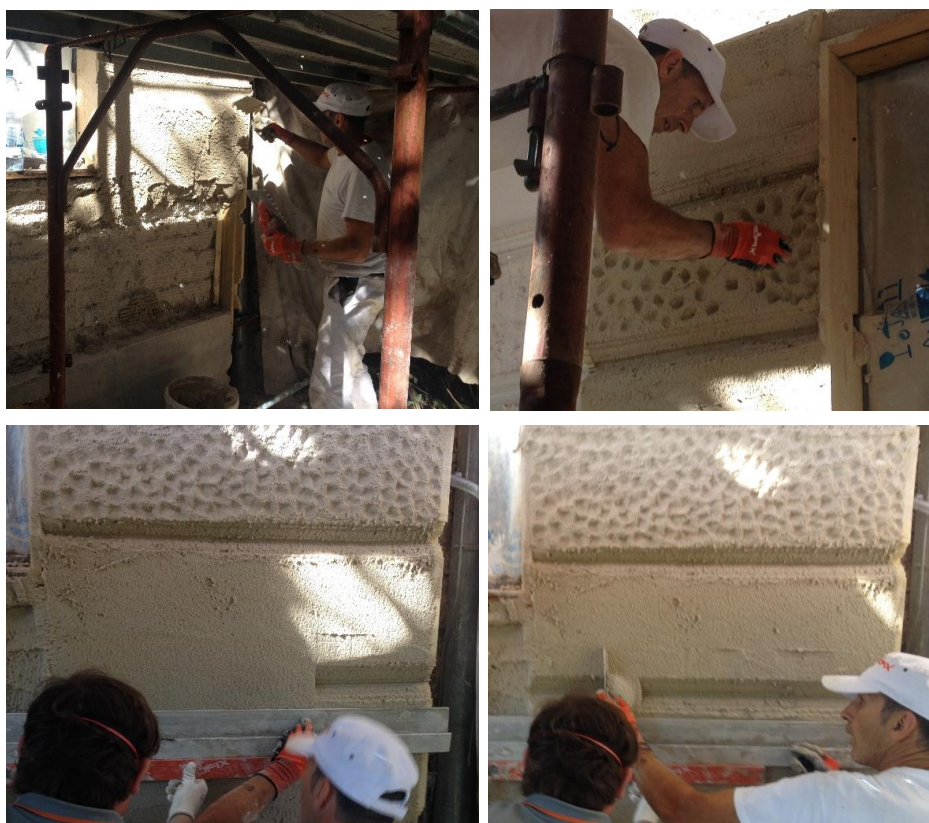
Figure 3. Stepwise application of the aerogel-based rendering without reinforcement mesh to an external façade, and processing to mimic decorative elements of the original façade. A clear indication for its advantageous high workability.
