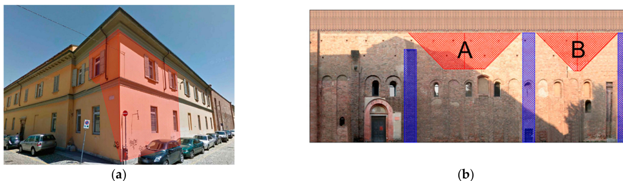
Figure 9. Identification of the possible overturning mechanism of the façade involving portions of the orthogonal walls at more than one storey (a). Definition of the constraints and possible activation areas of the out-of-plane two-way bending mechanisms (b). (Photos taken by the authors).
