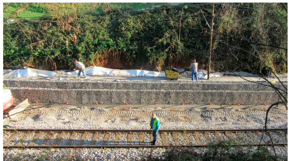
Figure 3. Compacting the last layer of the composite.
