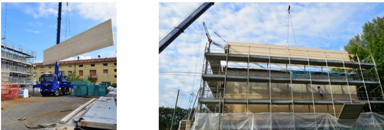
Figure 15. Details of the prefabricated structural intervention under construction.
