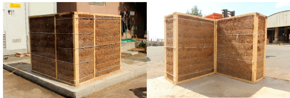
Figure 4. Construction of a prototype wall for the validation of the constructive process: view of the corner from the outside (image on the left) and the inside (image on the right).
