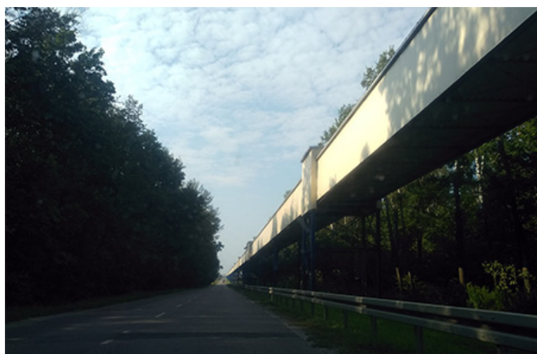
Figure 3. Overground belt flyover located by the road in the Puchaczów commune.
