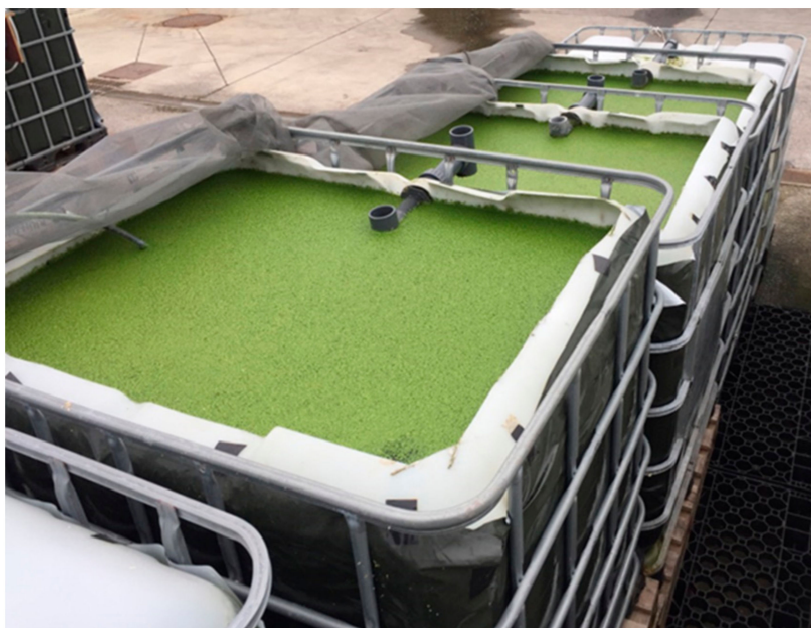
Figure A1. Above, a schematic representation of the cubicontainer cascade. From left to right, the medium was pumped with a flow pump (D) from the influent storage cubicontainer (A) into the second cubicontainer (B.1). By gravitational forces, the water flowed down the cubicontainers cascade and was stored in the effluent storage cubicontainer (C). The duckweed was grown on the cultivation cubicontainers (B.1; B.2; B.3). Picture of the running cascade containing the reference medium is shown below.
