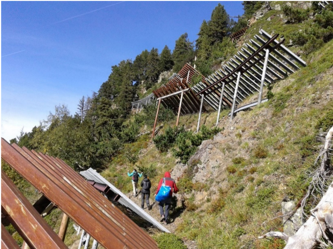
Figure 1. Anti-avalanche structures in Thiel corridor above Barèges.
