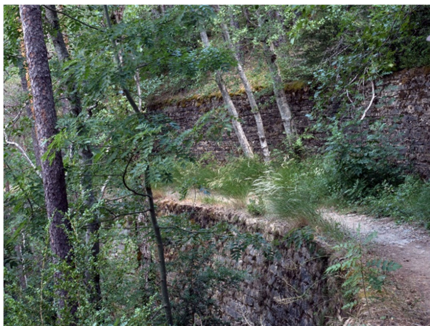
Figure 4. Stabilization terraces in the Arratiecho watershed.
