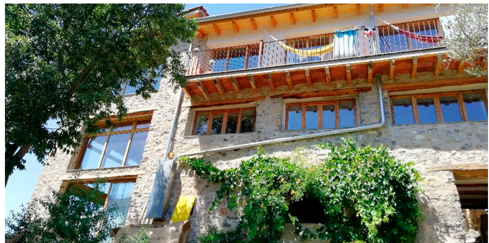
Figure 4. View of the south-facing façade of the case-study building.
