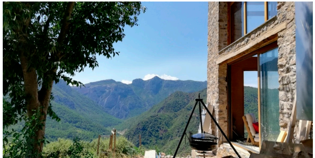
Figure 3. Exterior view of the case-study building.
