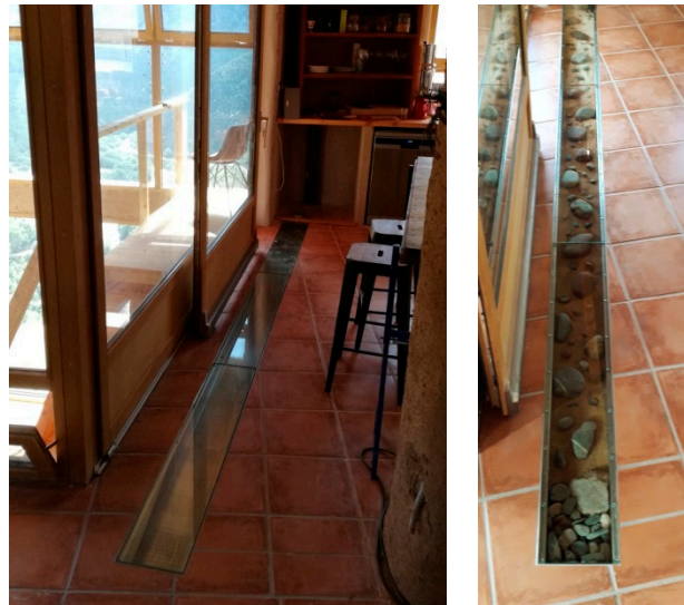
Figure 10. The Interior river channel.
