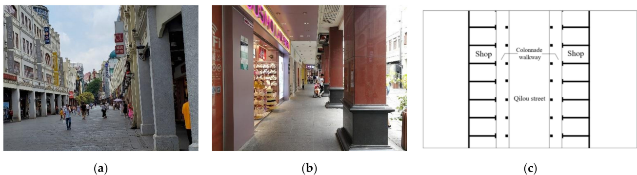
Figure 1. Traditional block in Nanning: (a) qilou shopping street; (b) colonnade walkway of qilou street; (c) layout of shops.
