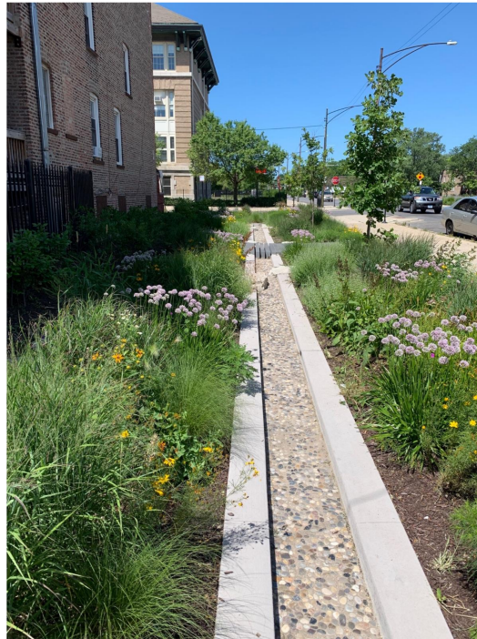
Figure 9. Resilient Corridor stormwater street-level feature, Chicago. Photo by Michael Berkshire.
