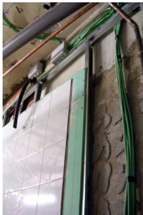
Figure 2. General view of today's wall lining system at a work site.
