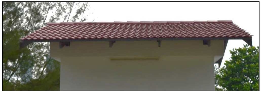
Figure 8. Red roof of Test Cell A.
