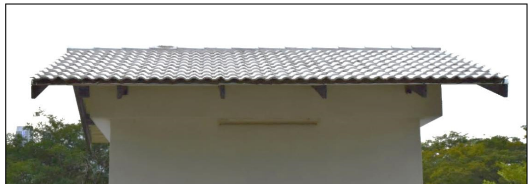
Figure 9. White roof of Test Cell B.
