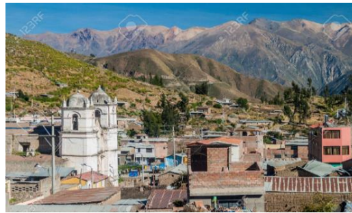
Figure 4. SCENARIO B—CABANACONDE: the use of industrialized techniques without technical assistance does not guarantee the structural safety of the houses, in addition to irreversibly damaging the urban image. ©Matyas Rehak.
