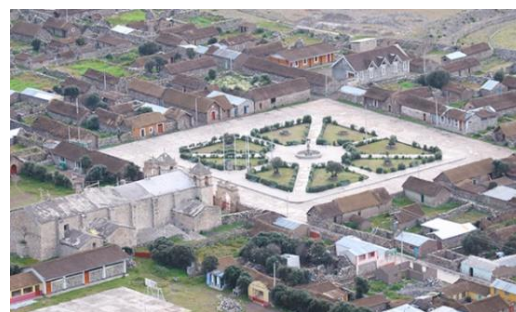
Figure 3. SCENARIO A—SIBAYO: with the use of traditional building techniques and technical assistance, safe homes were constructed, becoming a prominent tourist attraction in the Colca Valley.
