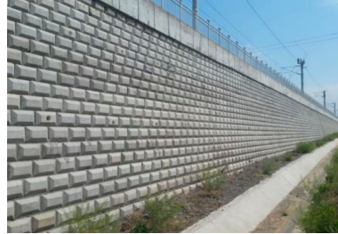
Figure 1. Modular-reinforced earth-retaining wall of Qingrong Intercity Railway.
