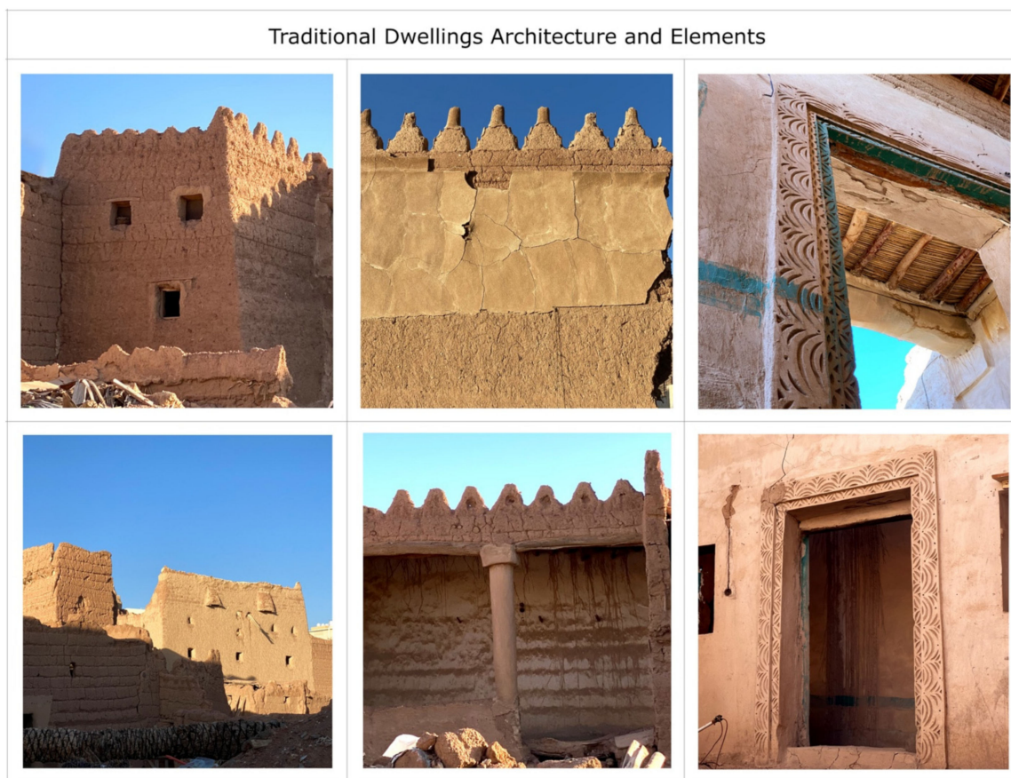
Figure 8. Several architectural elements, textures, and decorations in the traditional Hail City dwellings.
