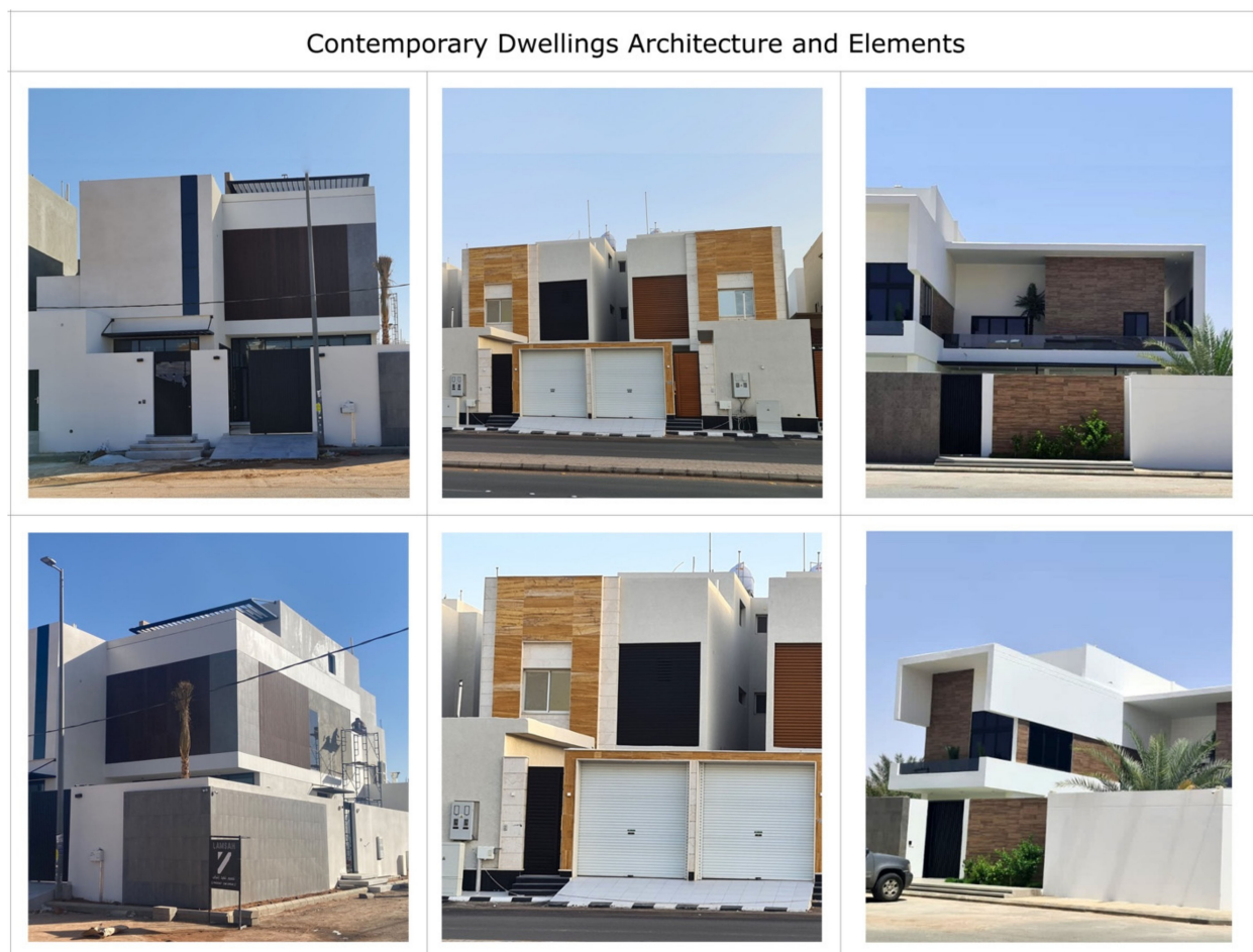
Figure 21. Several architectural elements, textures, and decorations from “Contemporary” Hail City dwellings.
