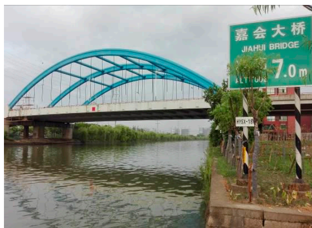
Figure 4. Elevation photo of Jiahui Bridge.
