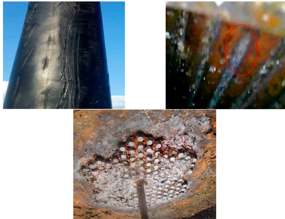
Figure 5. Pulling sling damage condition diagram.
