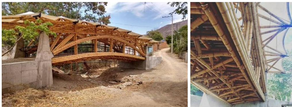
Figure 1. Low-traffic bamboo bridge (source: Authors).
