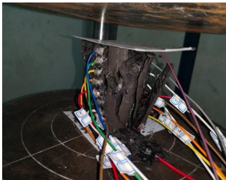
Figure 11. Photograph of sample M-3 after damage.
