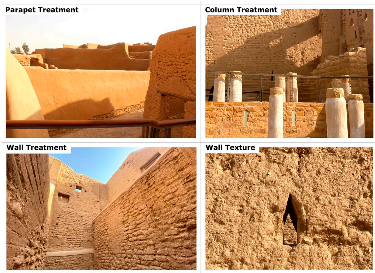
Figure 10. Samples of At-Turaif conservation treatment and construction. Source: Authors.
