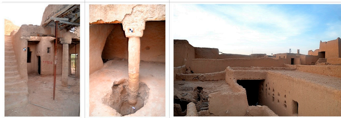
Figure 7. Example of the building restoration and rehabilitation process. Source: Authors.
