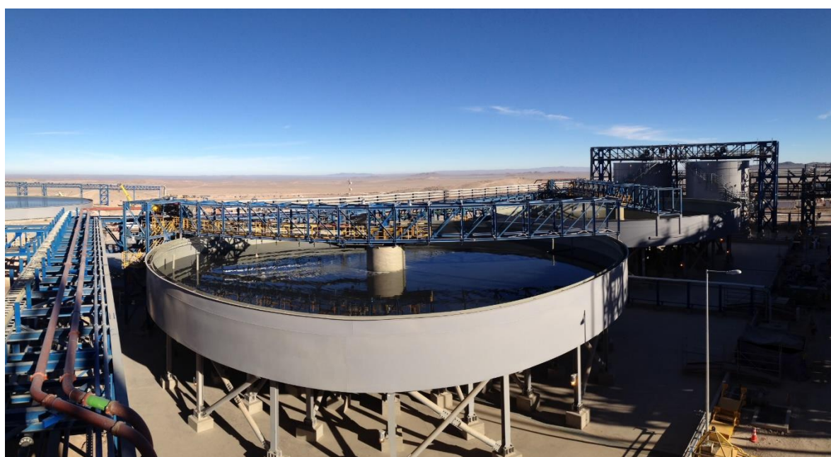
Figure 23. Thickening Process Plant in Sierra Gorda Mining Project.
