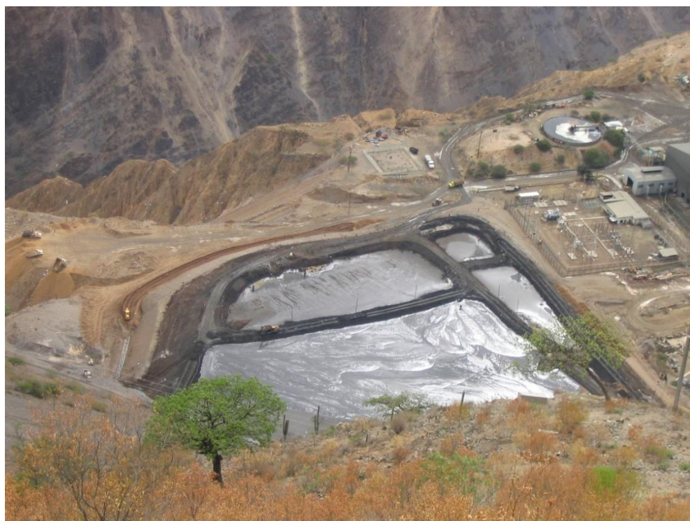
Figure 62. Cobriza Paste Tailings Disposal in Platanal TSF.
