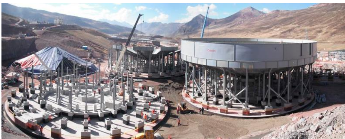
Figure 42. Tailings Thickeners under Construction—Toromocho Mining Project.
