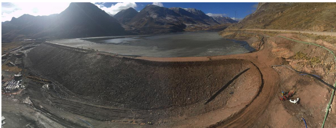
Figure 65. Typical Dam Crest View of Rumichaca Paste TSF.
