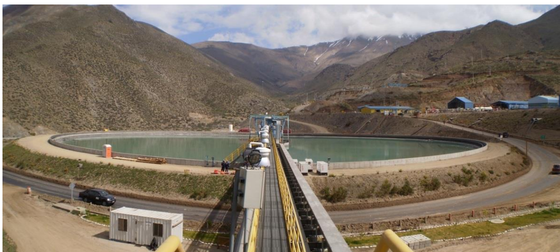
Figure 3. Tailings High-Rate Thickeners in Los Pelambres Mine—Chile.
