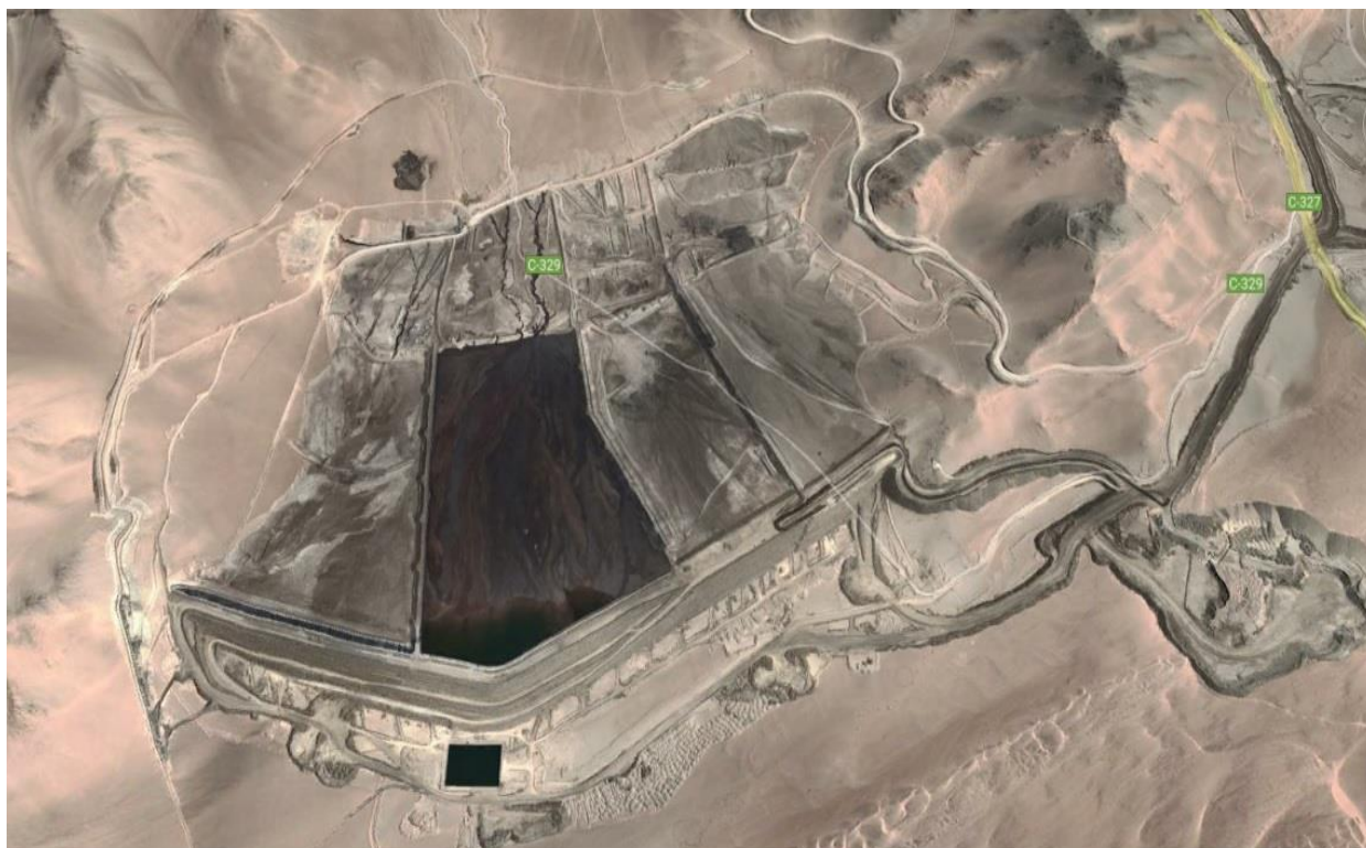
Figure 32. Los Corralillos Thickened TSF in Cerro Negro Norte Mining Project.
