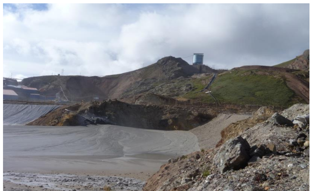
Figure 56. Paste Tailings Disposal—Chungar TSF.
