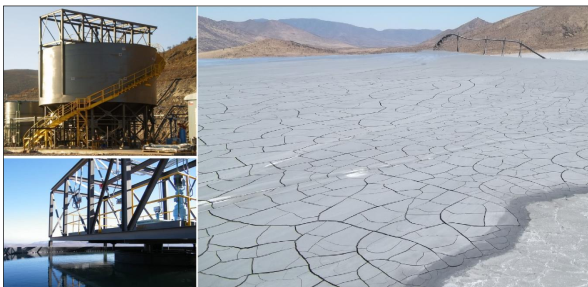
Figure 16. Delta paste tailings thickening plant and paste tailings disposal [5,36].
