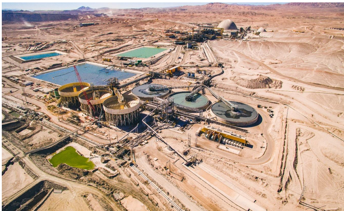
Figure 19. Thickening Process Plant in Centinela Mining Project.
