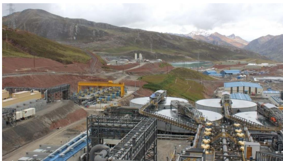
Figure 43. Tailings Thickening Plant and Positive Displacement Pump Station—Toromocho Mining Project.
