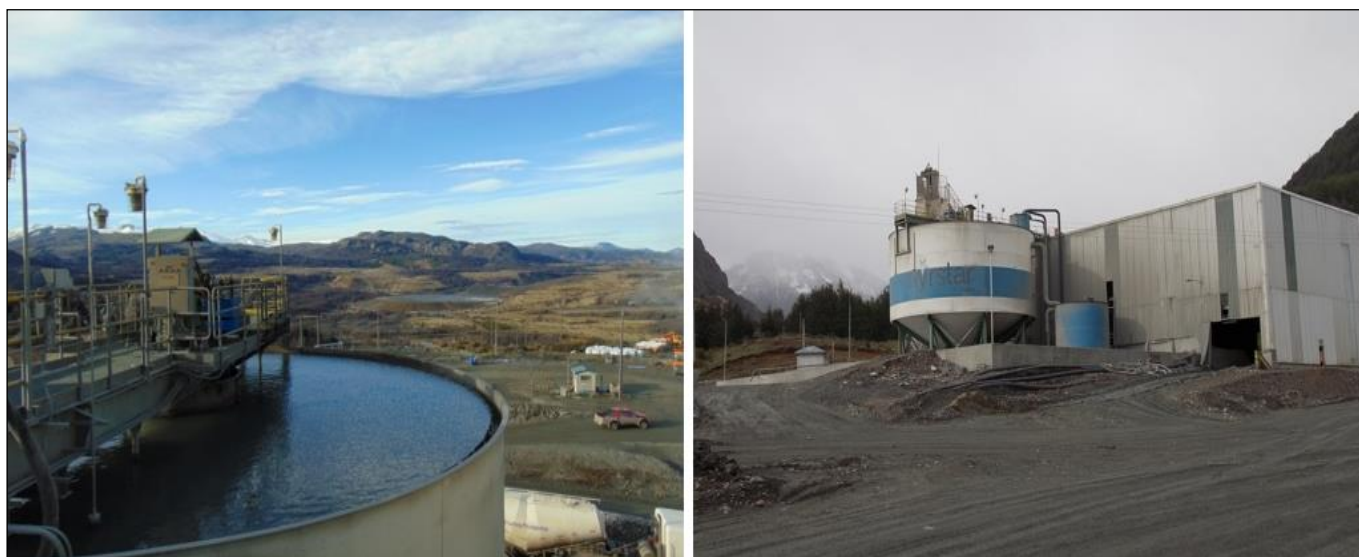
Figure 17. El Toqui paste tailings thickening plant [39,52].
