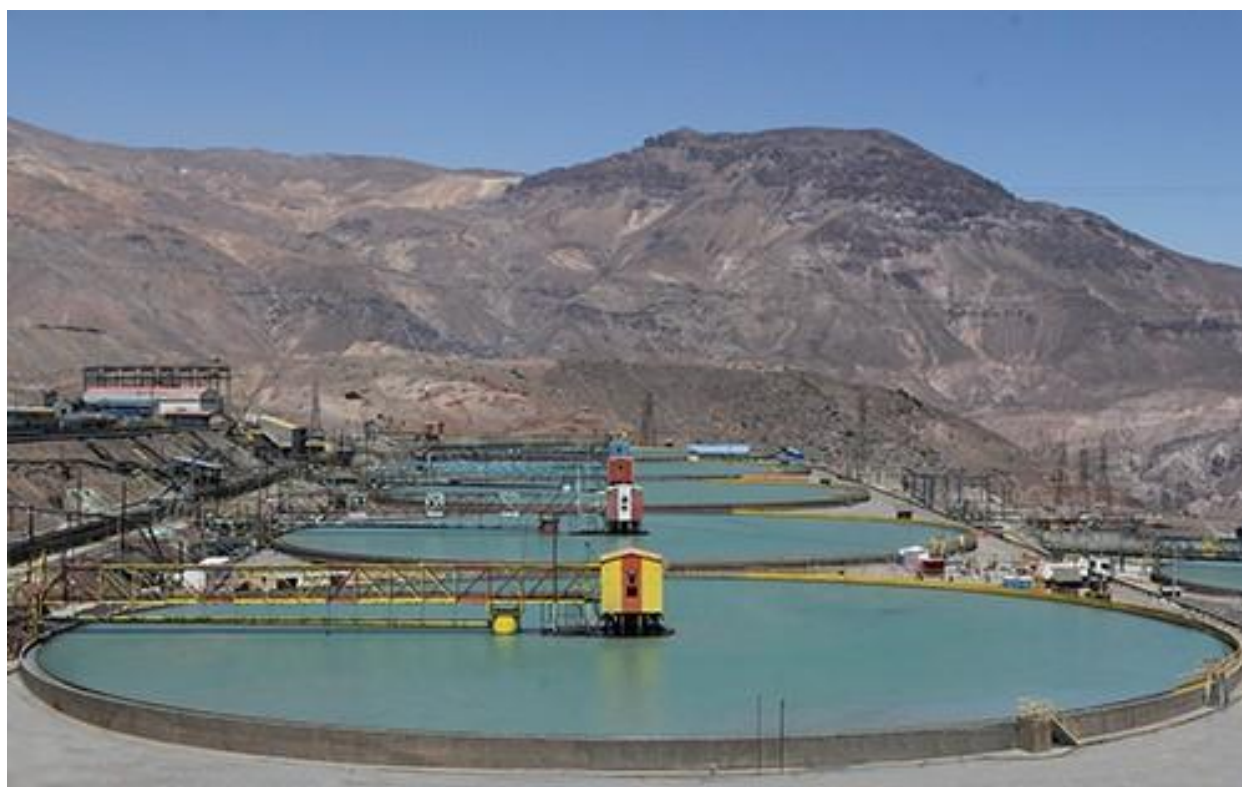
Figure 2. Tailings Conventional Thickeners in El Teniente Mine—Chile.
