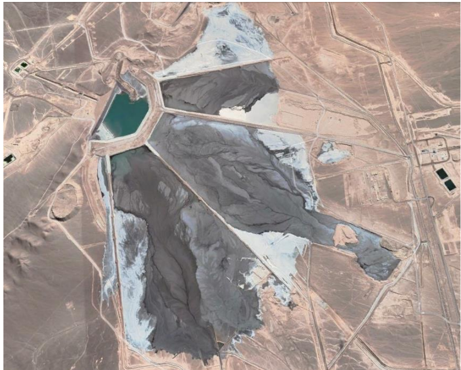
Figure 26. Layout View Spence Tailings Storage Facility.
