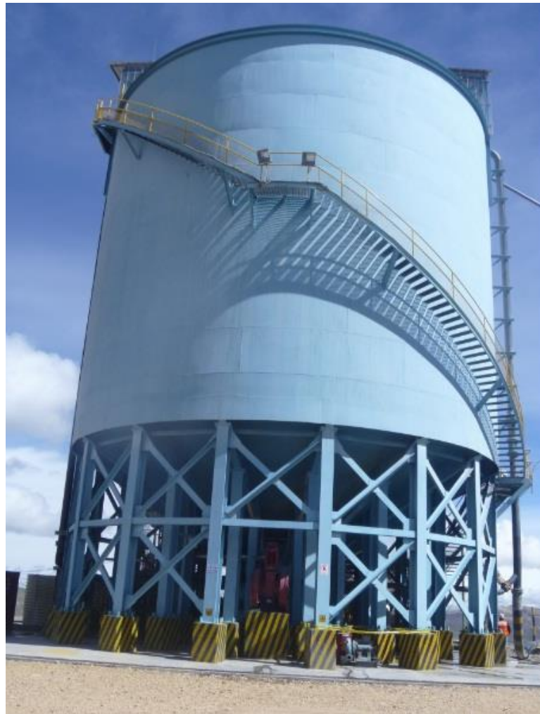
Figure 55. Deep Cone Thickener for obtain Paste Tailings—Chungar Thickening Plant.
