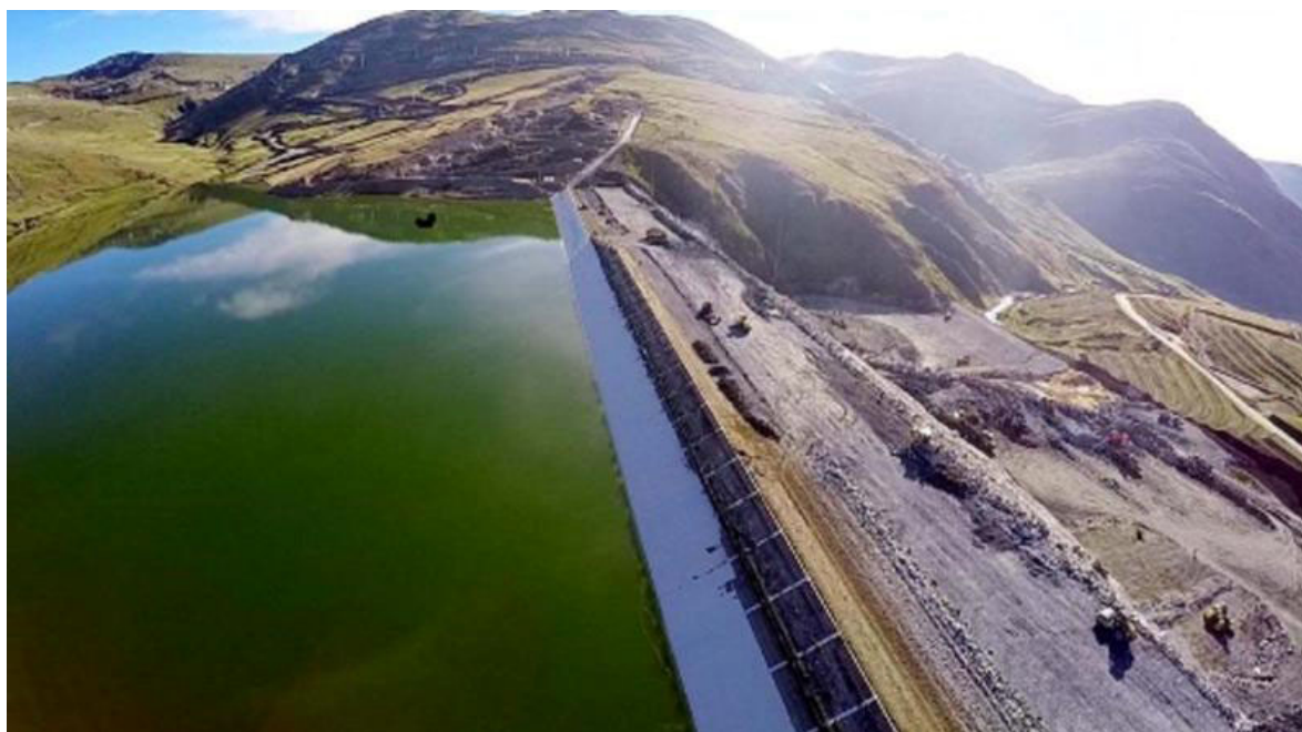
Figure 51. Dam Crest View of Las Bambas Thickened TSF.
