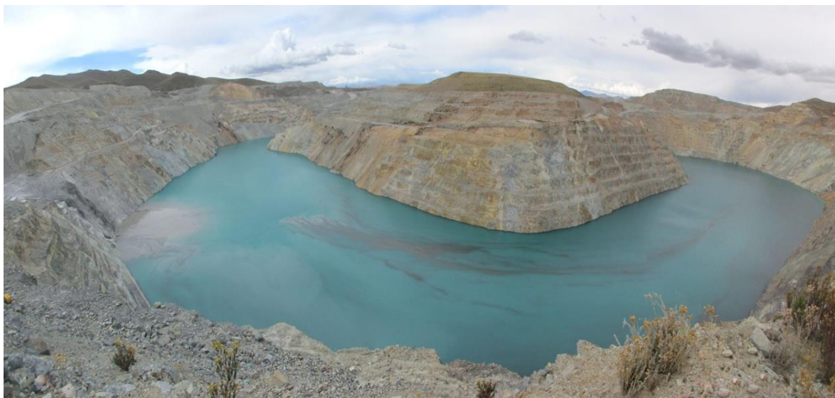
Figure 48. Tintaya Open Pit filled with Antapaccay Thickened Tailings.
