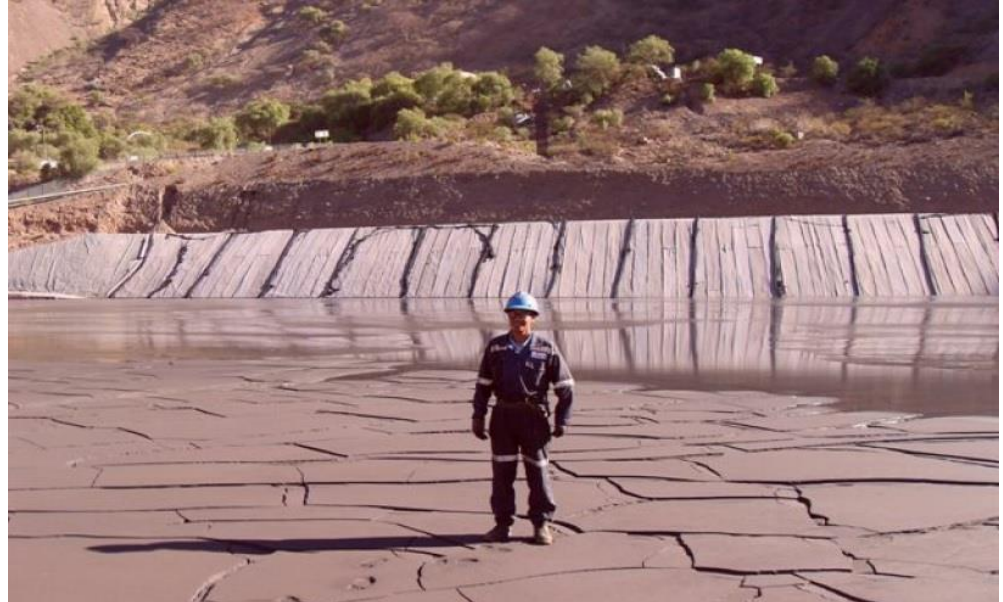
Figure 60. Cobriza Paste Tailings Disposal in Limonar TSF.
