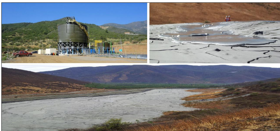
Figure 15. Las Cenizas DCT overview and paste tailings disposal at TSF [36,51].
