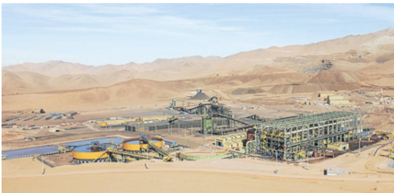
Figure 30. Tailings Thickening and Pumping Station—Cerro Negro Norte Process Plant.
