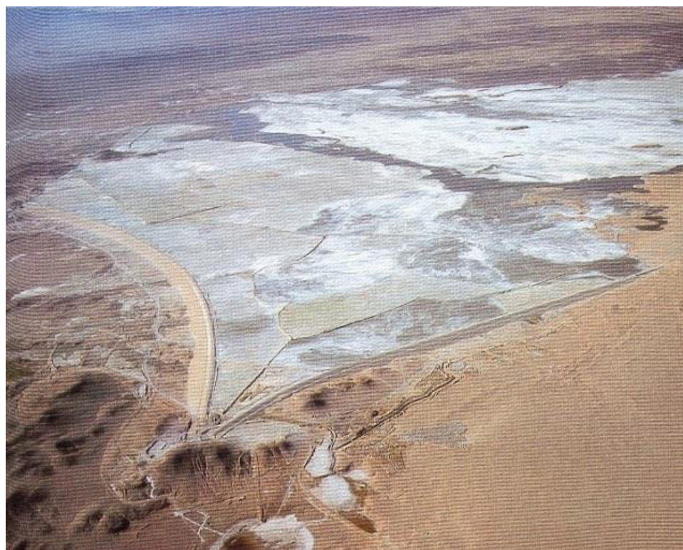
Figure 28. Panoramic View of Talabre Tailings Storage Facility.
