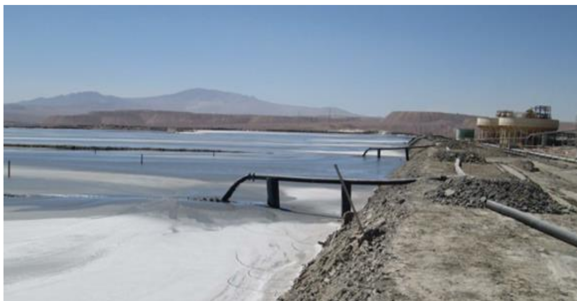
Figure 20. Thickened Tailings Discharge in Spigots in Centinela Mining Project.
