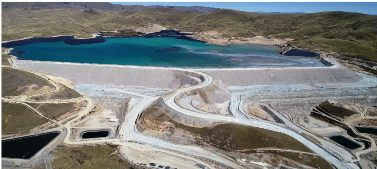
Figure 54. Front view Constancia Thickened TSF Mine Waste Rock Dam.
