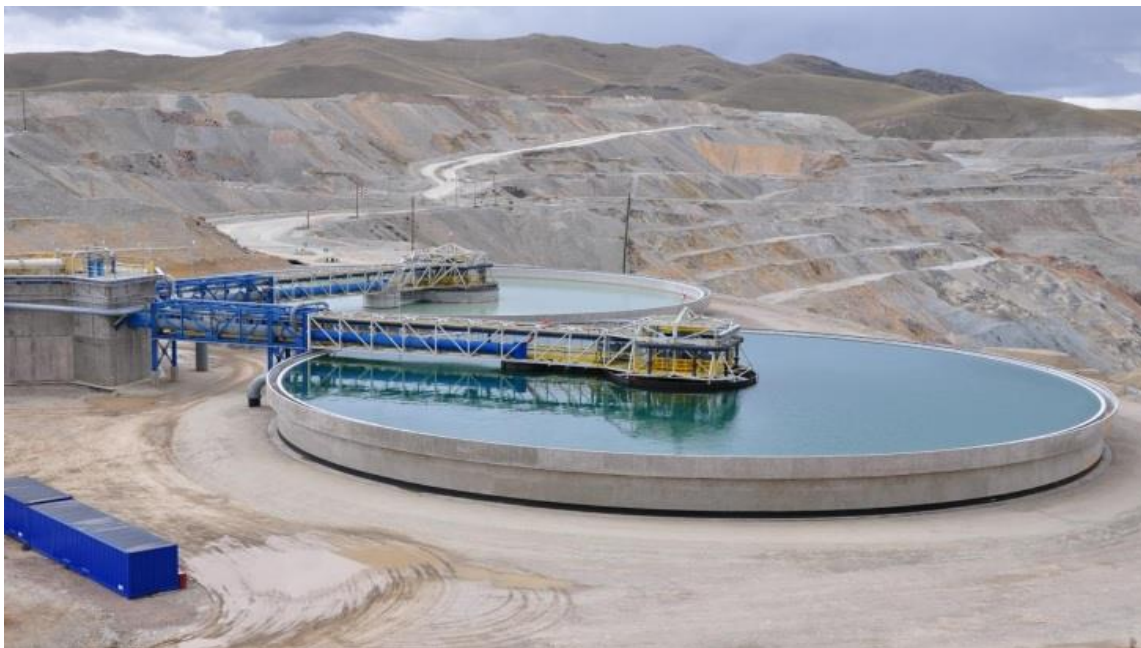
Figure 47. Antapaccay Tailings Thickeners Located Close to Tintaya Open Pit.
