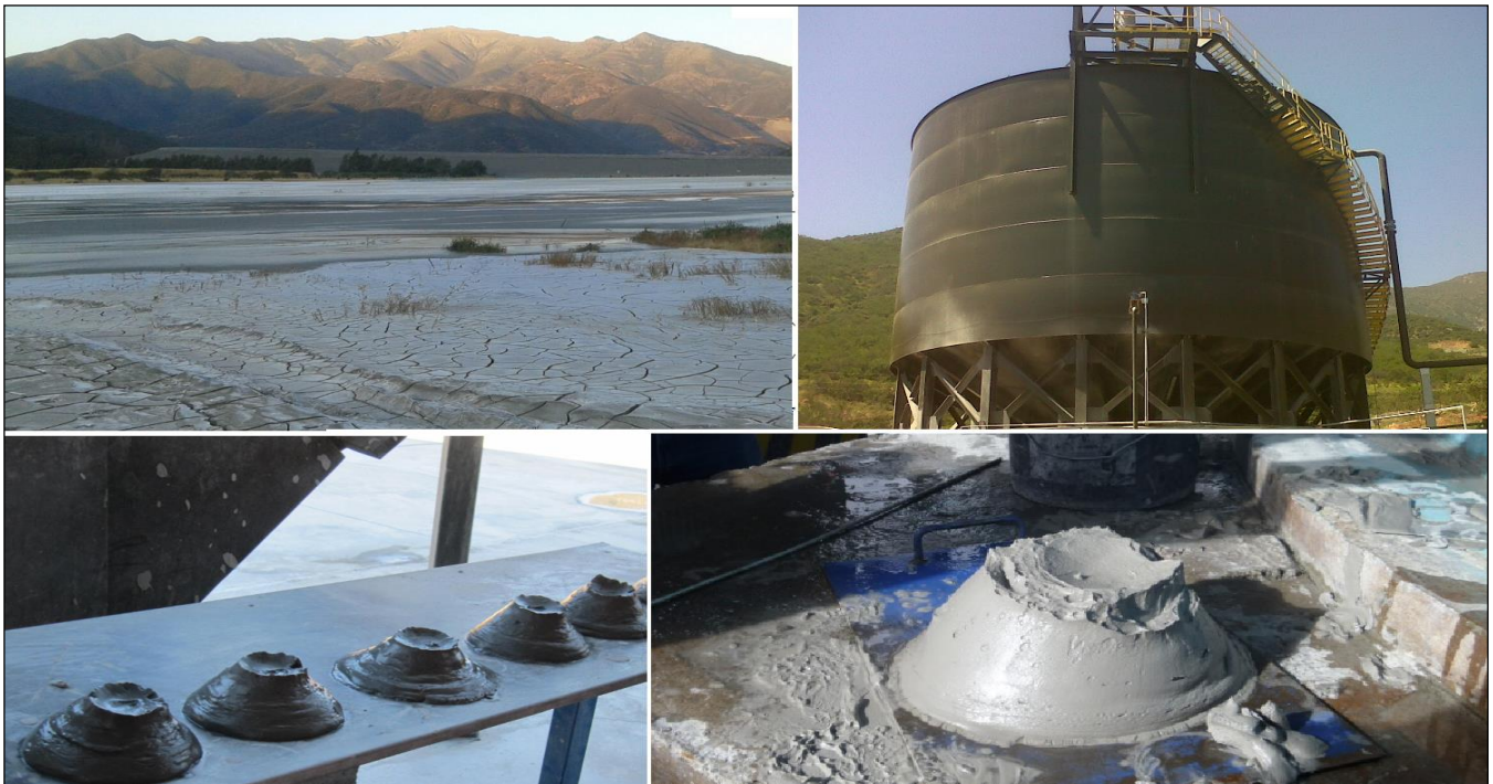
Figure 18. Alhué paste tailings thickening plant and paste TSF [38].
