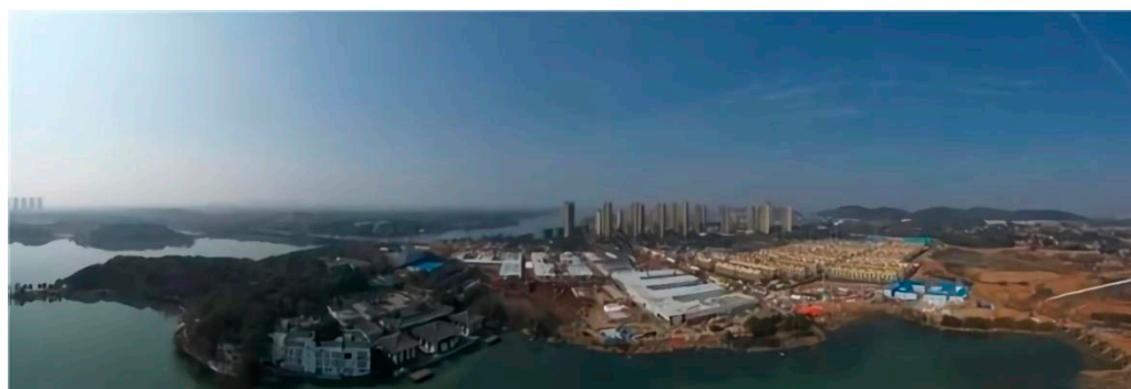
Figure 2. Panoramic view of emergency hospital construction.
