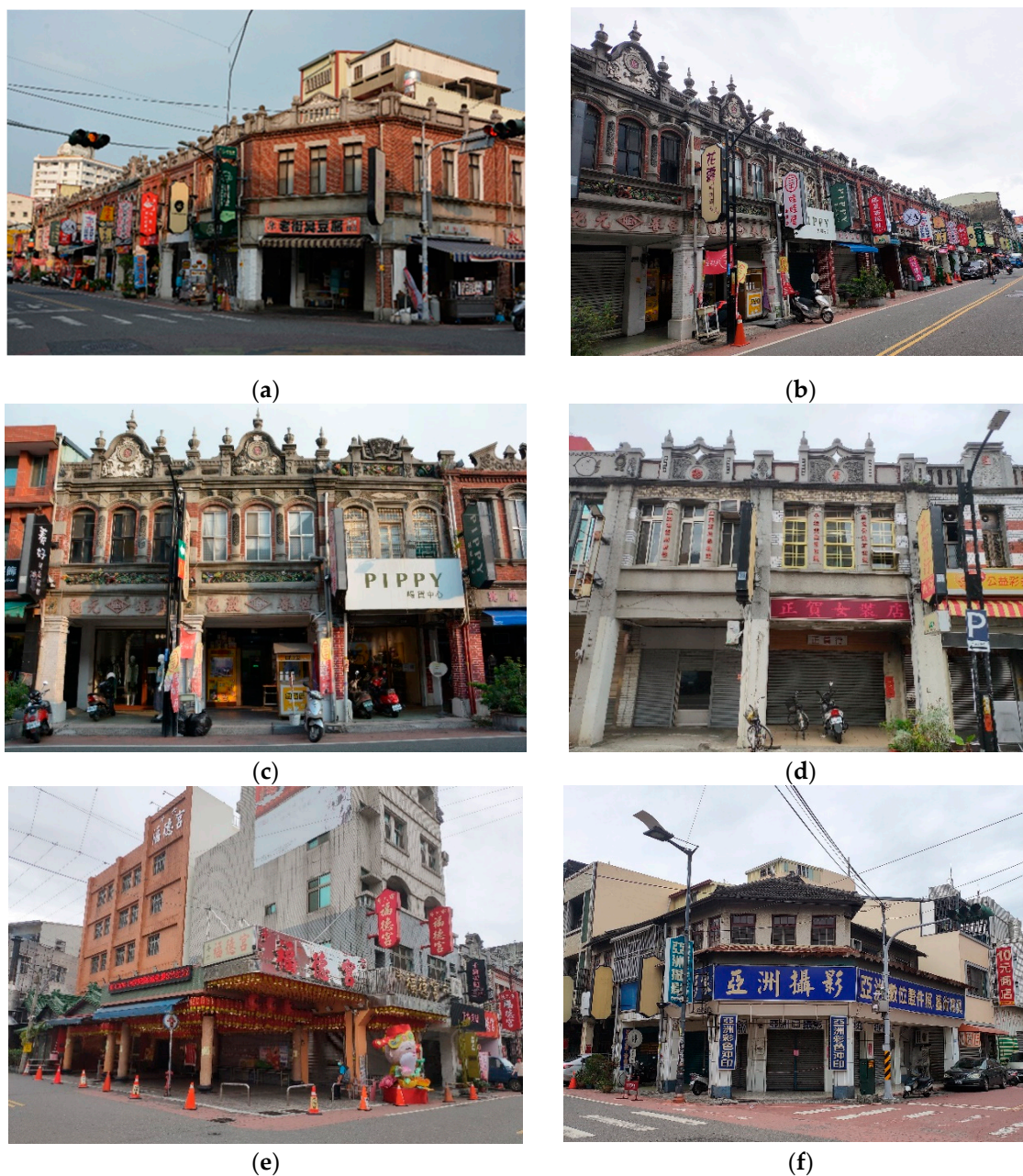
Figure 2. Building landscape of Taiping Old Street. (a,b) Street houses. (c) Baroque-style street houses with traditional Chinese patterns. (d) Street houses integrated with Roman pillars and traditional Chinese couplets. (e) Fude Palace (a temple for worshipping the local God of the Land). (f) Street house in Japanese style.
