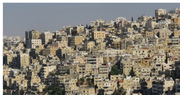
Figure 16. Preserving the contours maintained the city's original character. Source: The Author.
