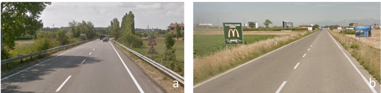
Figure 3. Photos of SR206: 33 + 700 km southbound (a), and 39 + 200 km northbound (b).
