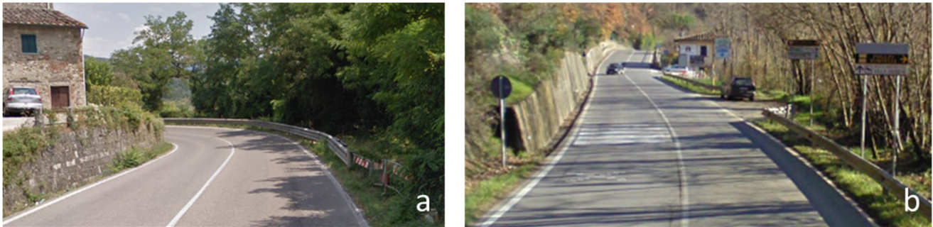
Figure 2. Photos of SR2: 282 + 100 km northbound (a), and 288 + 400 km southbound (b).
