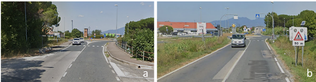
Figure 12. Approach to roundabout: SR206_031_4 (a) and SR206_032_1 (b).
