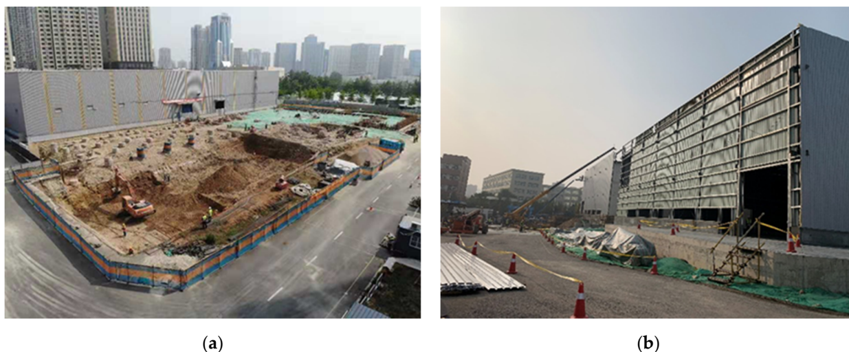
Figure 4. New warehouse project of Siemens: (a) Before construction; (b) after construction.
