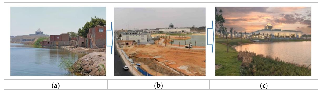
Figure 4. The renovation phases of the NMEC: (a) the site was turned into an informal area, (b) during construction, (c) the museum site after development in Al Fustat, Cairo.
